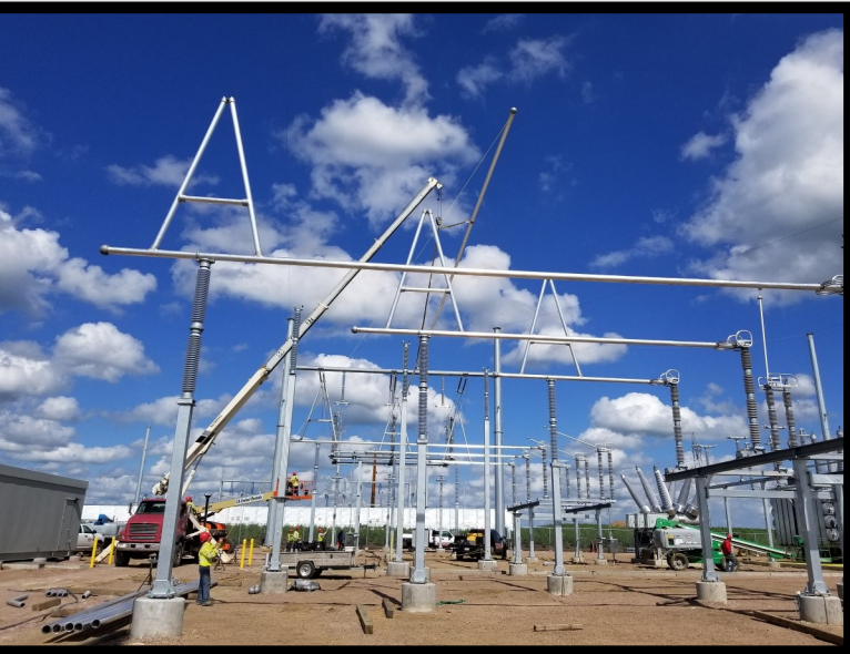
Various installation of the bus system. Quite a bit of the bus (both rigid and flexible) was able to be pre-fabricated in Rapid City. It was then hauled to the site where final assembly and installation took place.
