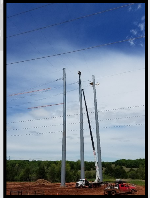
Installing Pilot Line over two 345 kV
