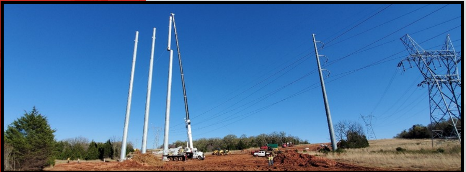
Utilizing all 197' of boom on the Tadano to set the 187' 3 Poles
