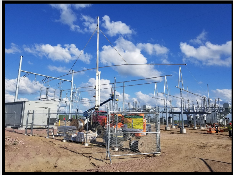
Various installation of the bus system. Quite a bit of the bus (both rigid and flexible) was able to be pre-fabricated in Rapid City. It was then hauled to the site where final assembly and installation took place.
